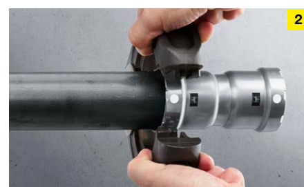
For pressing Megapress S connectors from 1 ¼ inch upwards, only press rings with hinged adapter jaws are used. For smaller sizes between ½ and 1 inch, both press jaws and press rings with hinged adapter jaws are available.
